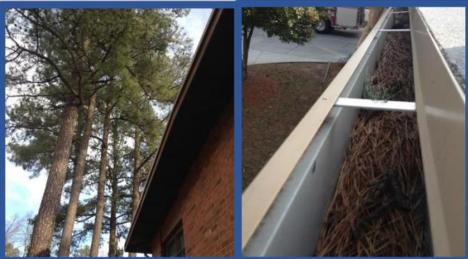
Overhanging vegetation, as seen on the left, can lead to debris in the gutters which will reduce the flow of water to the rainwater storage tank and decrease the quality of the harvested rainwater.
